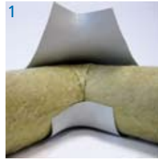
Fitting of a premoulded bend
